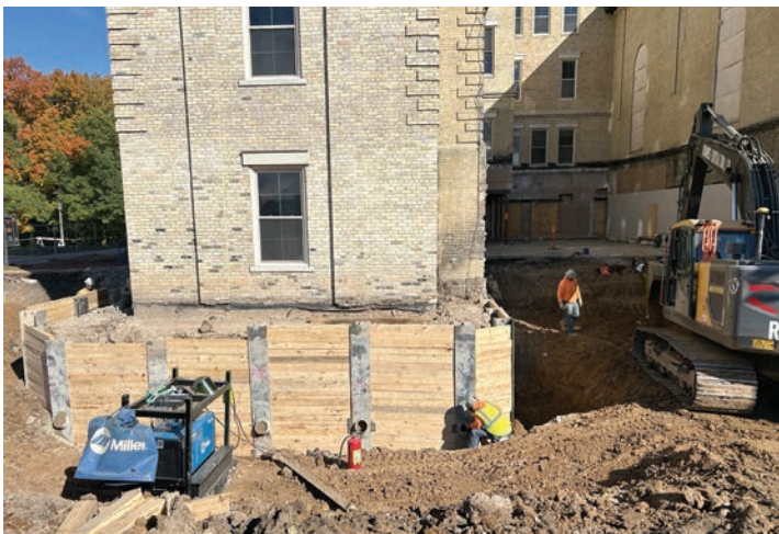
H-piles are in place to shore up the foundation before the expansion begins.
